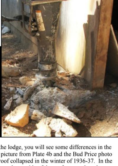
In the photo below, the 1960's earthquake retrofit footings that were installed by Ben and Butch Filer are getting a new bigger and complementary design.
