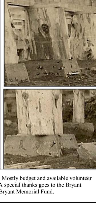
Unfortunately, erosion has undercut the footings at the front of the lodge. The poles and posts reinstalled during the 60's have also rotted away and the need to get the Lodge ready for the next 75 years (not to mention to bring it up to code) has brought us to that point in time where we have to replace the last 14 footings around the main hall.
