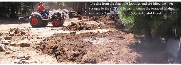
You now see the outline of the dedication center taking shape. To the outside of the rocks now holding the dirt in place, we will be pouring a concrete 18" retaining wall for the Scout Law display. In front of the Scout Law wall, there will be a 4' skirting that will help keep the dust down and allow for a "Buy a Brick" to help fund the renovation of camp.
